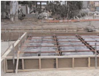
throughout the footprint area. A five inch post-tension reinforced concrete slab is then monolithically poured, the Waffleboxes allowing for any expansive soil movement. The pour also creates concrete beams running through the footprint and perimeter.
