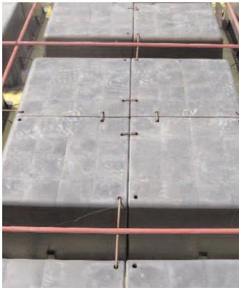
friendly"). The Wafflemat is created by connecting a series of Waffleboxes together, and evenly spacing them throughout the footprint area. A five inch post-tension reinforced concrete slab is then monolithically poured, the Waffleboxes allowing for any expansive soil movement. The pour also creates concrete beams running through the footprint and perimeter.
